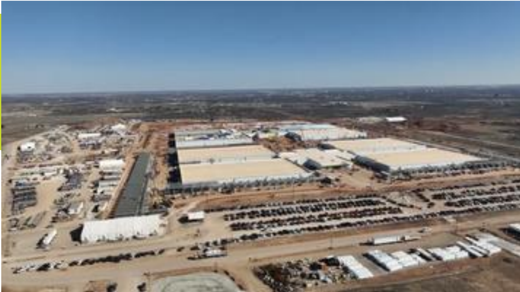
OpenAI Stargate facility in Abilene, TX (Data Center Dynamics)
