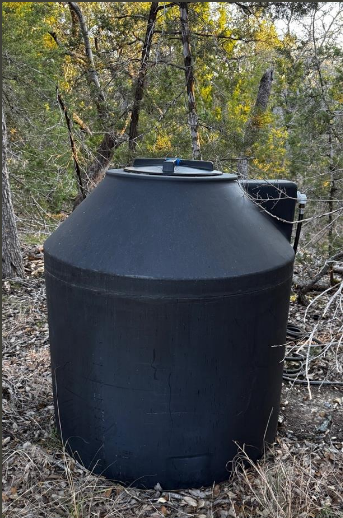
Recycled flush water
